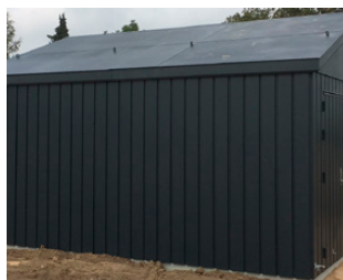
ZINC MAGNESIUM FACADE WITH PITCHED ROOF
