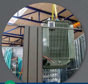
The secondary substation can be delivered as a Plug & Play solution, where the station is lifted with a concrete foundation on-site and placed upon a sand pad. The station is then connected, upon which it is operational. Readings are organised either by you or by Priess A/S.
